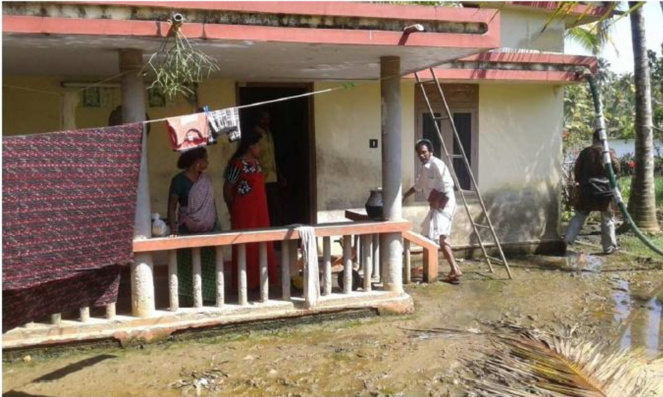
Photo 1: A residential building settled nearly 40cm in Kidapuram South. The stagnant water after high tide is seen on 23 rd February 2015. Note that the steps at the entrance have settled into the soft clay.
